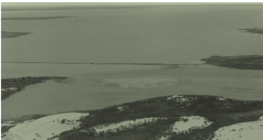
Tauwitchere Barrage no.(1) (2004)
