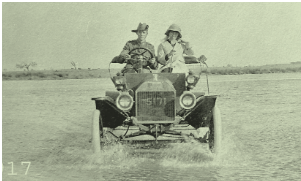
Flooded road Narrung District 1917
